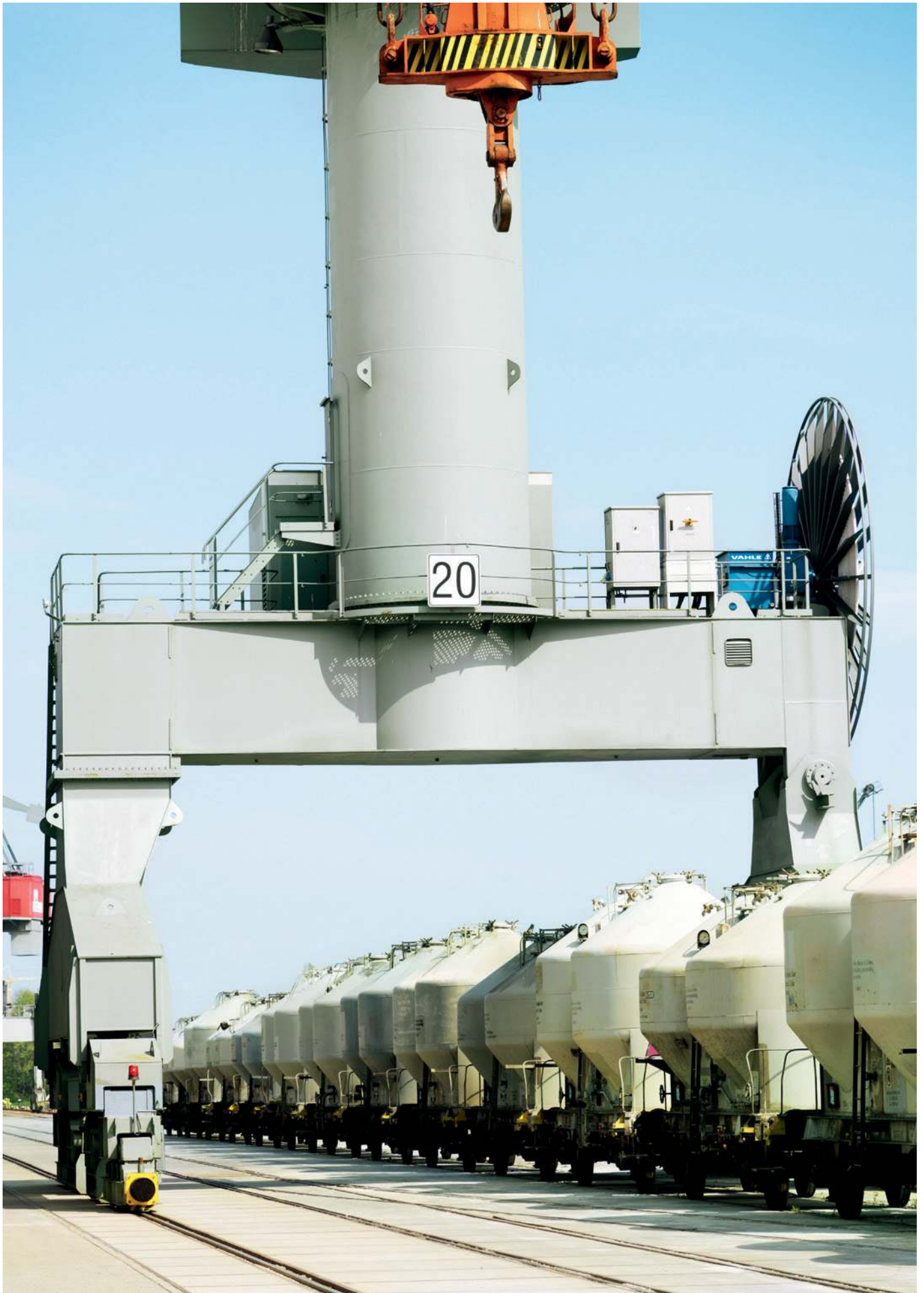
↑ Gantries present no obstacle to traffic
