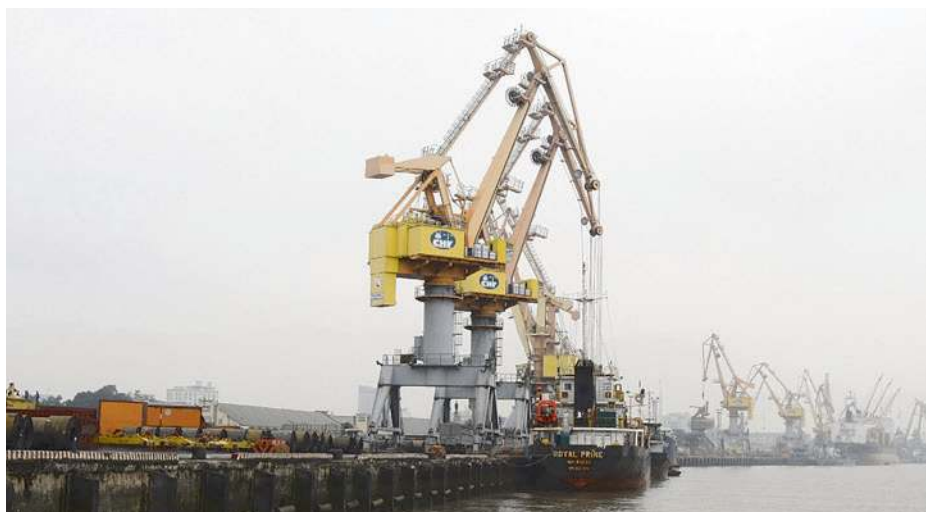
↑ Port companies in Haiphong/Vietnam rely on Tukan cranes
