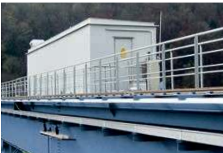
↑ The entire control system is installed in the electrocontainer to make maintenance easy
