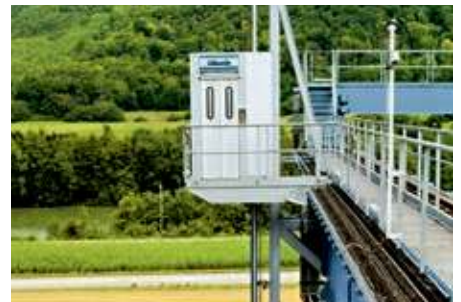
↑ Access – stairs, platforms, ladders and elevator
