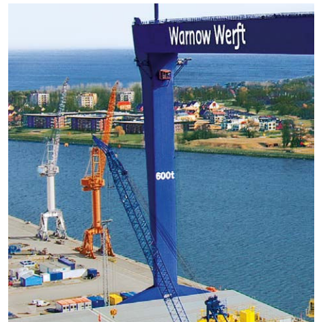
↑ Fixed Leg with Stairs and Elevator
