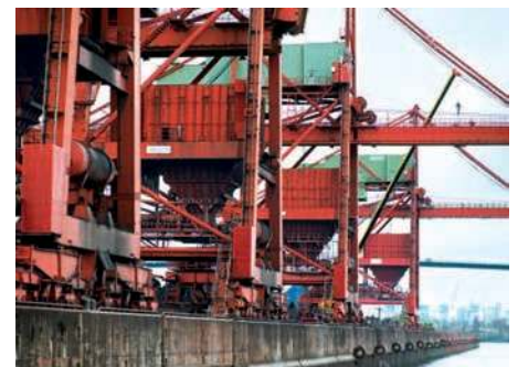
↑ Location of hopper next to vessel
