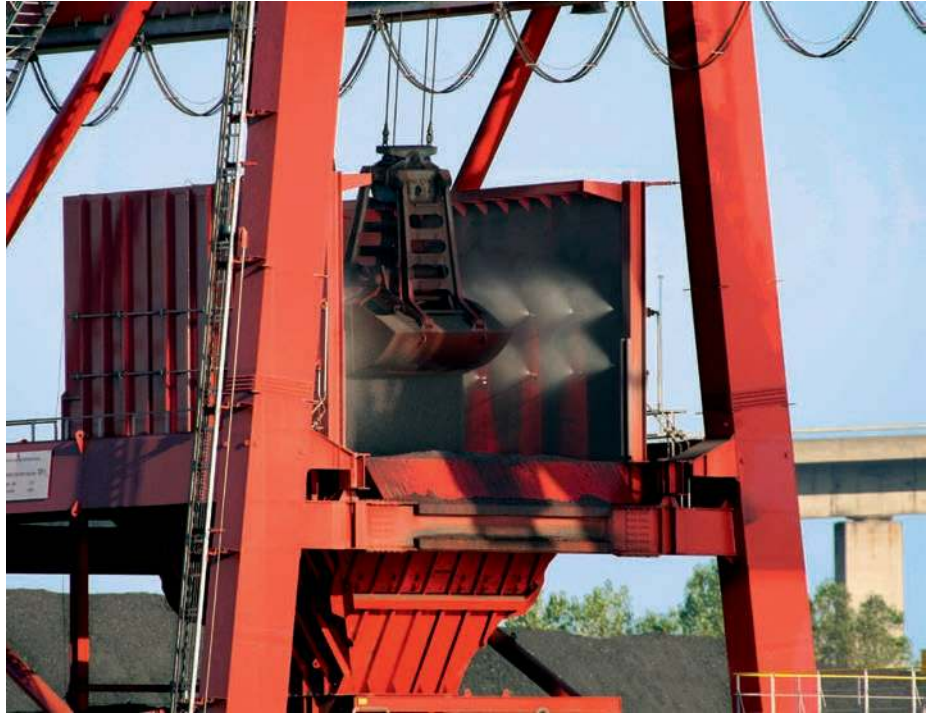
↑ Grab inside dust house with activated spraying system
