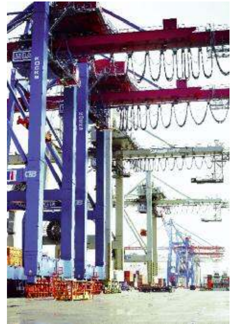
↑ Gantry structure with inside elevator and stairs
