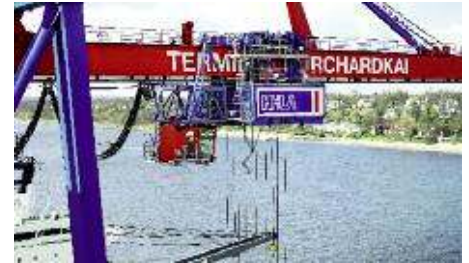
↑ Machinery house trolley on mono-box boom
