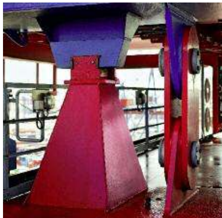
↑ Boom connection to the gantry at landside
