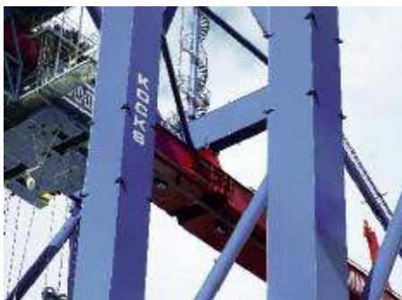
↑ Mechanical lock between waterside and landside boom
