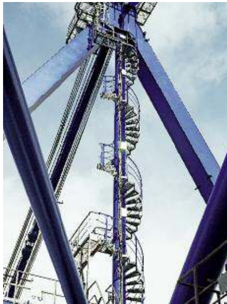
↑ Ascent platforms at pylon
